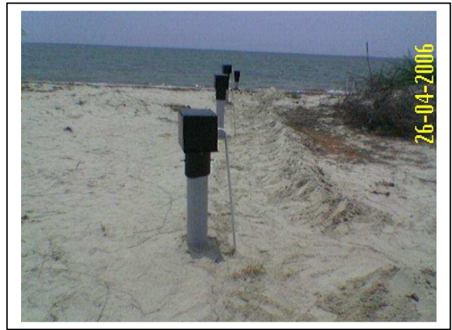
Array of 15 borewells in which the float sensors are introduced and connected to the 15-channel Water Level Recorder.
